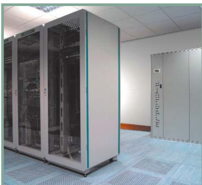
Data centre cooling
